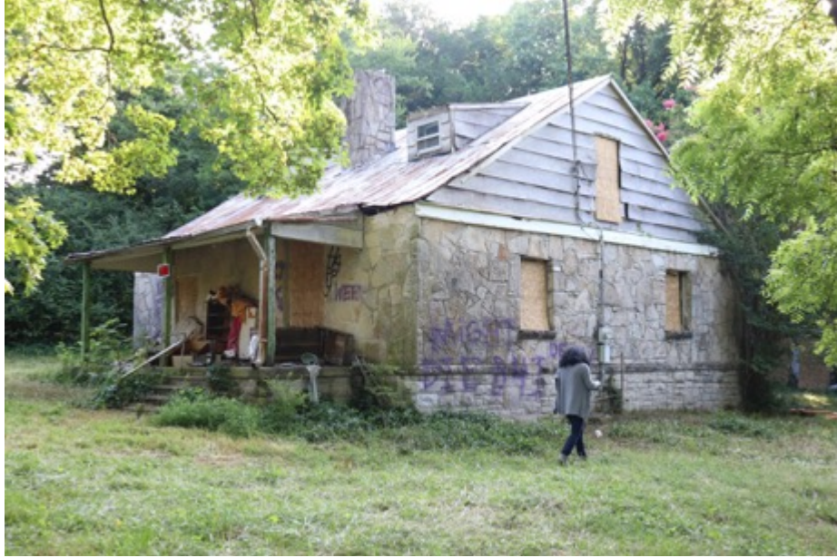
Figure 23. South Elevation. Cracks in exterior walls, wall tagged with graffiti, deteriorated fascia, and deteriorated synthetic gable siding. Photo taken July 2019.
