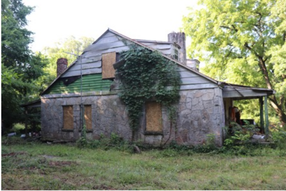
Figure 25. North Elevation. Deteriorated and missing synthetic siding and damage from ivy growth. Photo taken July 2019.
