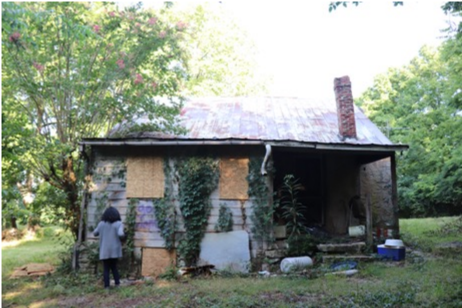
Figure 24. Rear of the house/East Elevation. Back porch has settled, deterioration of synthetic siding, and brick chimney causing a safety hazard. Photo taken July 2019.
