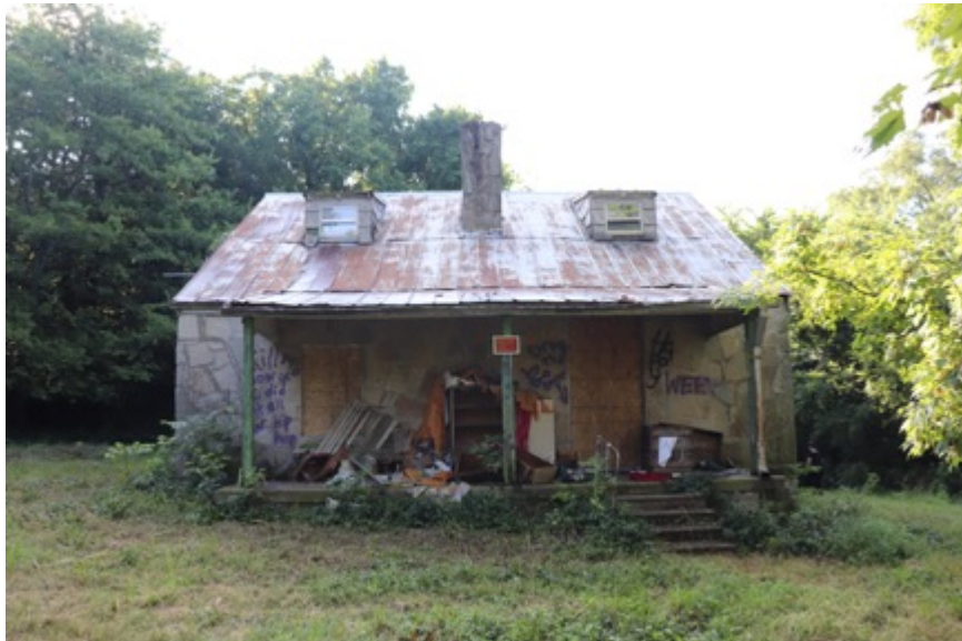
Figure 22. Façade/West Elevation. Porch has settled, walls tagged with graffiti, deterioration of roof, chimney is cracked. Photo taken July 2019.
